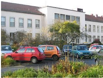
Picture 6: terrace side of the main building
